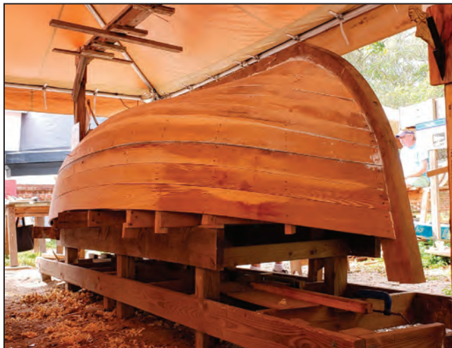
The skilled volunteer boatwrights of Heritage Boatworks at the St. Augustine Lighthouse & Maritime Museum put the final “whiskey plank” on a replica British yawl that they handcrafted over the past three years. The attachment of the last plank, technically called a shutter plan, earned the colorful nickname of “whiskey plank,” when boatwrights celebrated its placement with a “spirited” toast.
